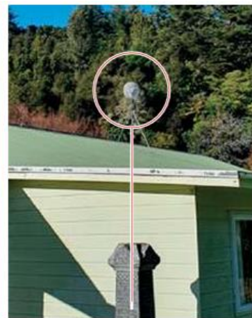
Marae rooftop antennae
